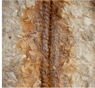
(b) Apparent rusty reinforcement in a structural element, with negligible reduction in the reinforcement section.
