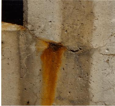
(a) Rust stain on a concrete structural element.
